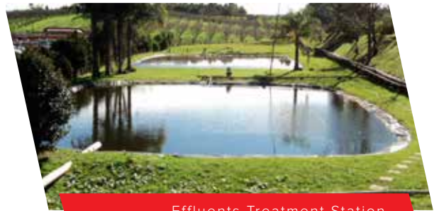
Effluents Treatment Station
