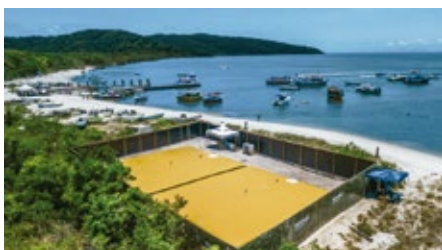
Flexible Tanks in the Ilha do Mel 300m 3 (Paranaguá / PR)
