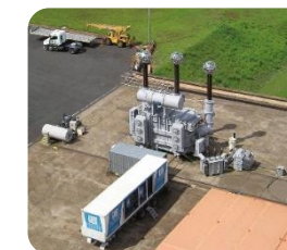
Retrofitting and Repowering Services Up to 550 kV
