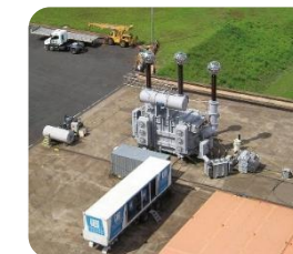
Retrofitting and Repowering Services Up to 550 kV
