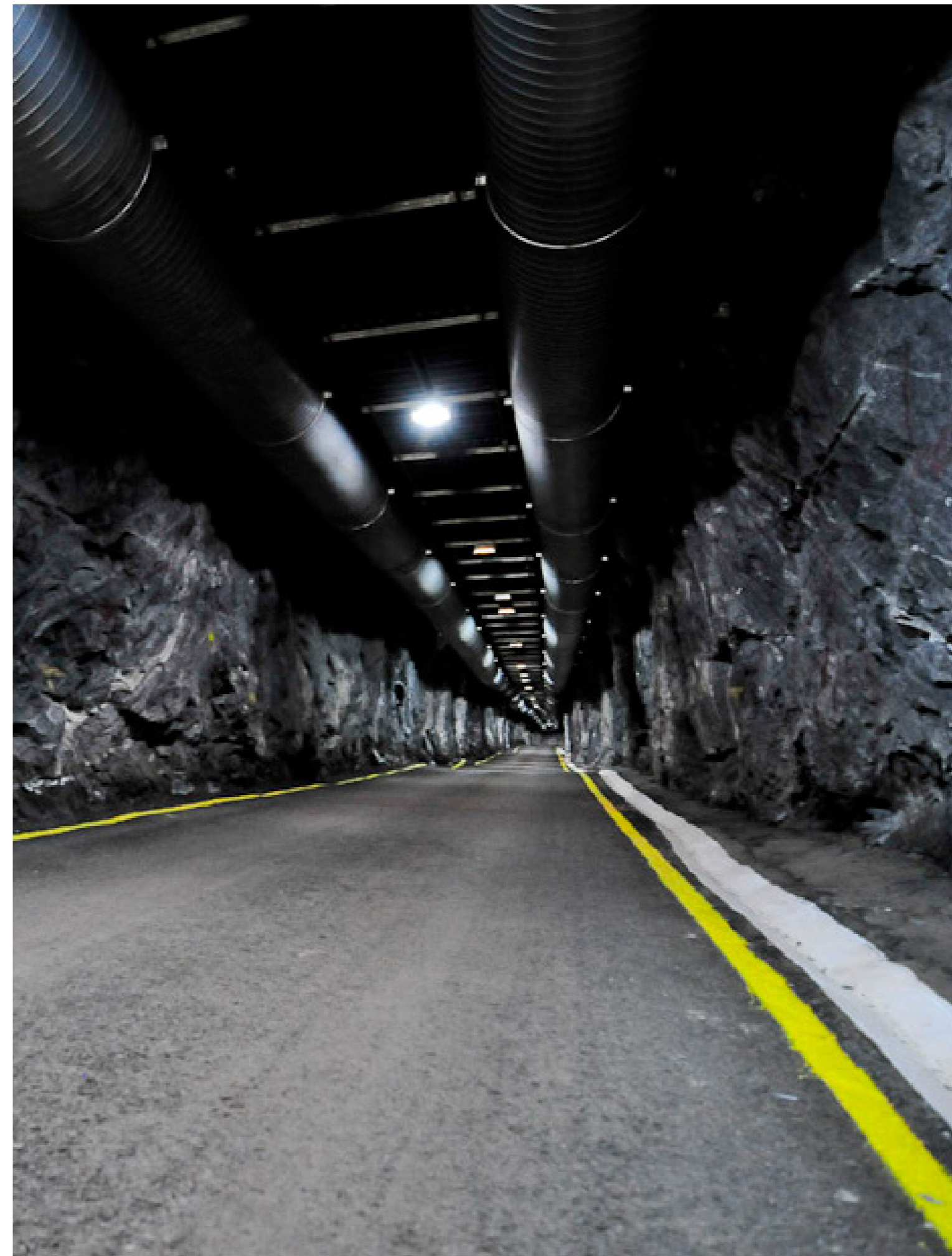
São João SMALL HYDROELECTRIC PLANT (ES)
